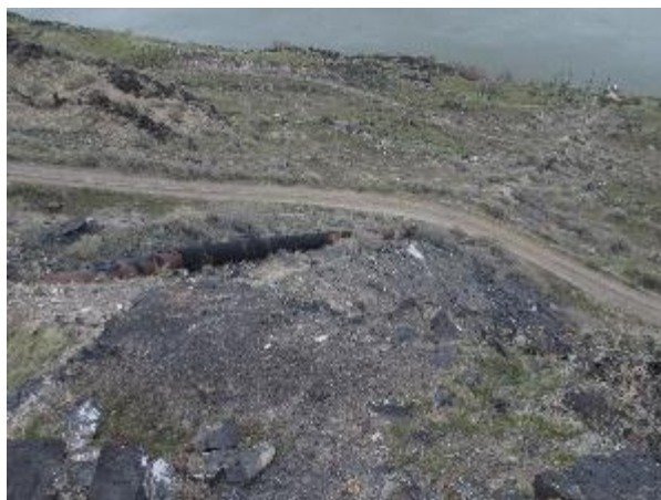
Western Alignment - existing pipeline and pump station from the rim above the project area.
