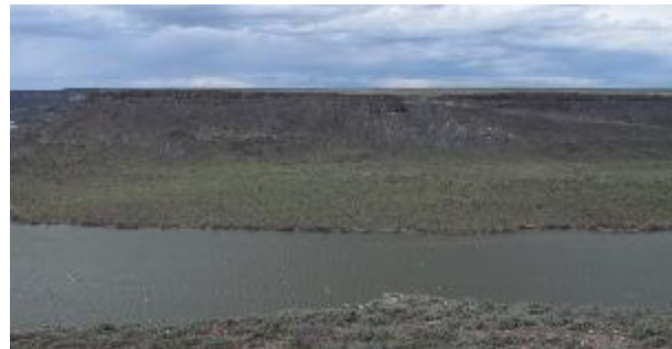
Eastern Alignment - view of the project location from the south side of the reservoir.
